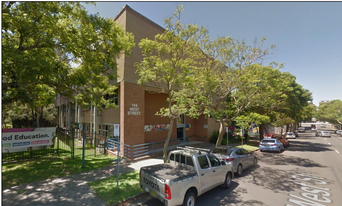
Figure 1: View of the site from the north west from West Street, Crows Nest
